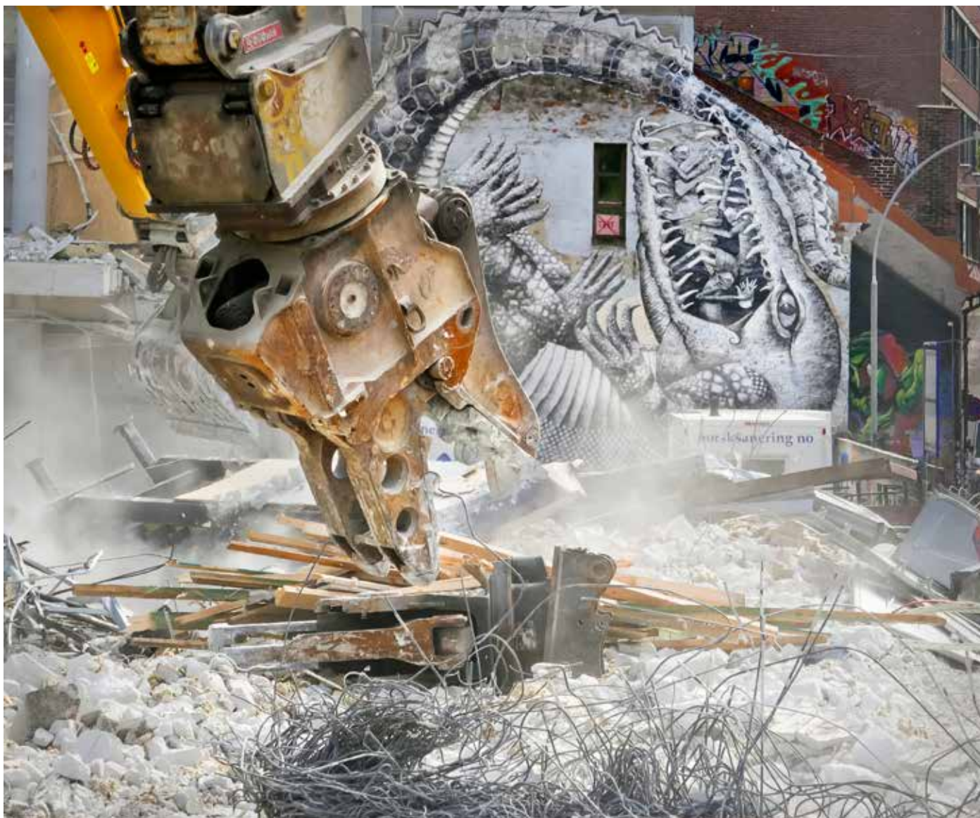
Above: Prehistoric Demolition, Oslo
