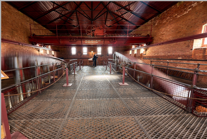
The engine beams working at Claymills pumping engines
